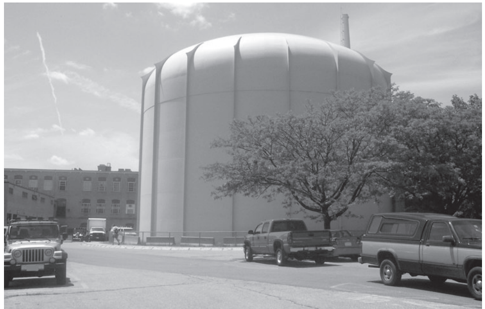
Figure 2: Research Reactor Building Surrounded by Jersey Barriers
